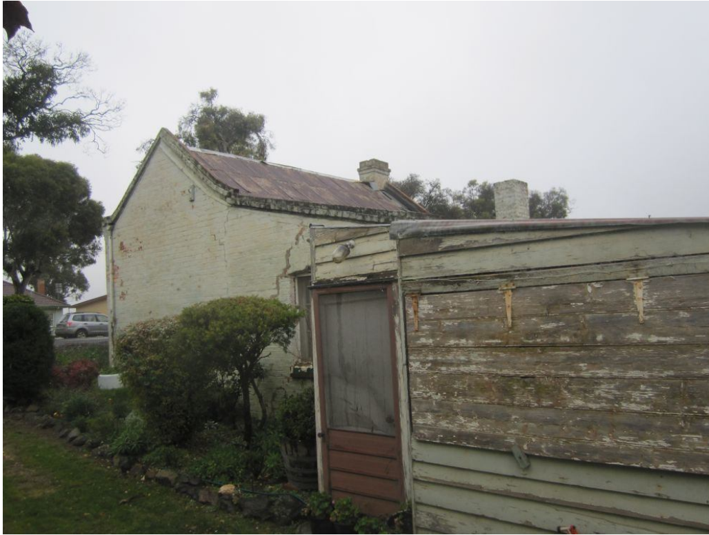
Figure 4 Rear view east side
