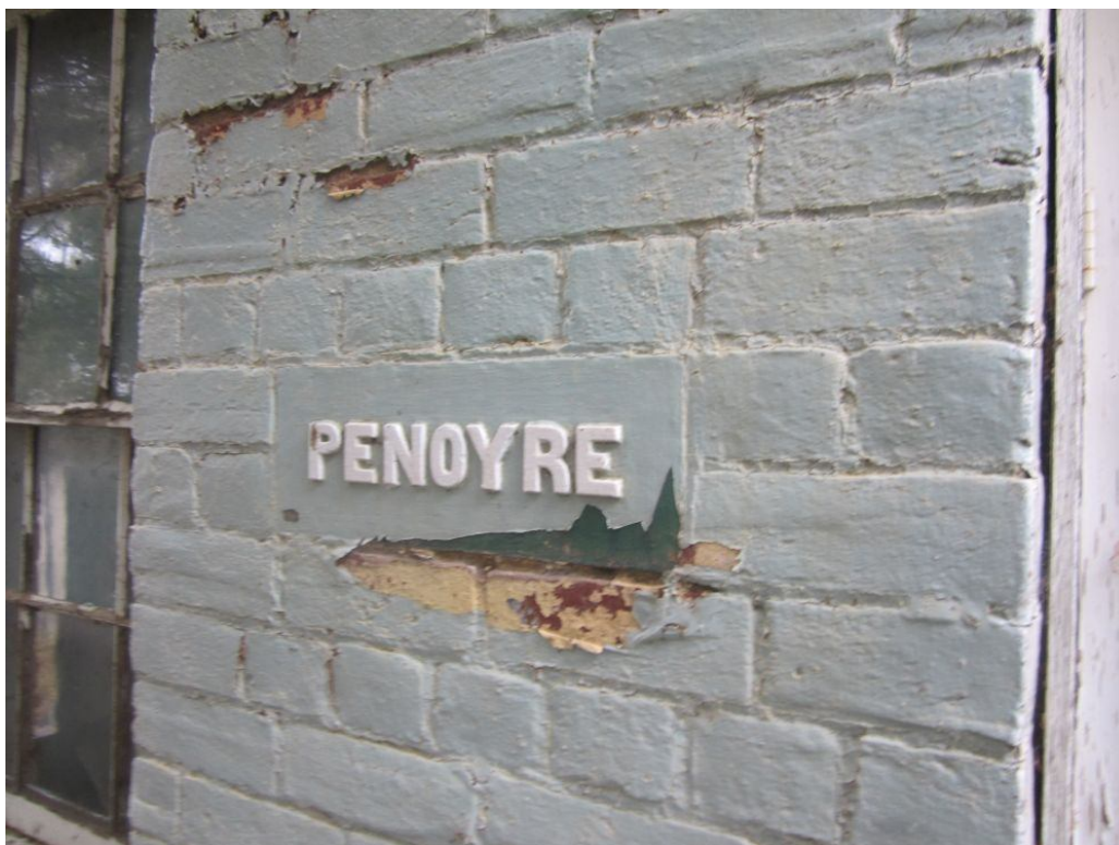
Figure 5 Name plate left of door note exposed brickwork below paint
