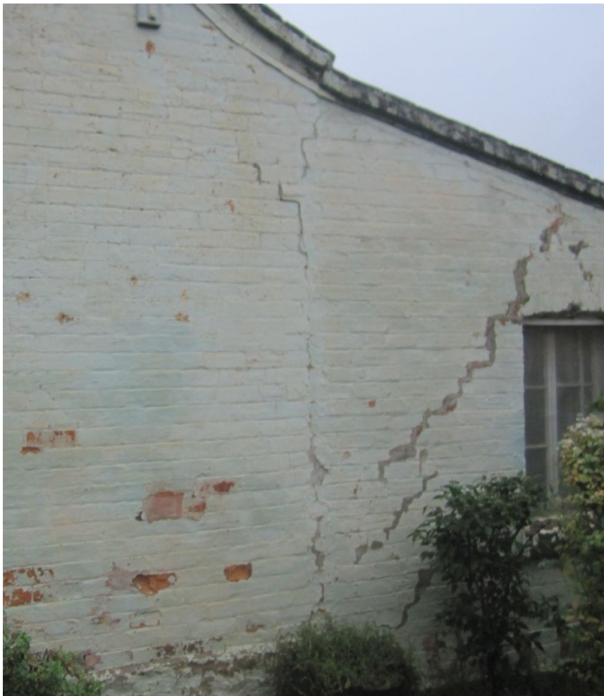
Figure 7 Connection between gable and skillion sections – note casement window
